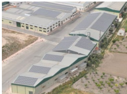
1 The 217-kilowatt facility in Valle Hermoso
