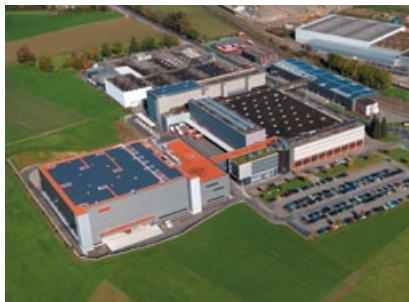
1 The 74-kilowatt facility in Adlisberg
